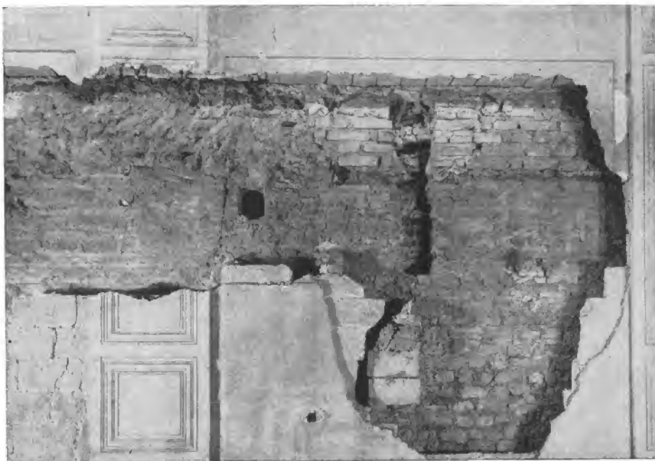
Fig. 43 — S. Lorenzo f.l.m. Soundings 1947-49. East basilica, south aisle, south wall, springing of entrance arch (Photo: Sansaini).
